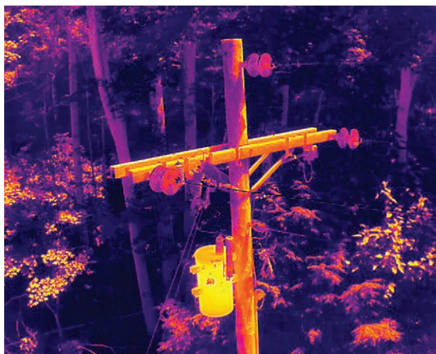
ASSESSING DAMAGE: Images from Somerset REC's drone help pinpoint equipment and infrastructure issues and enhance reliability for consumer-members.
